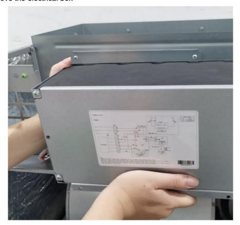
4. Disassemble the metal plate at the mounting hole of the electric heater
